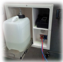
Ancillary equipment and peroxide container stored in the gas generator.
